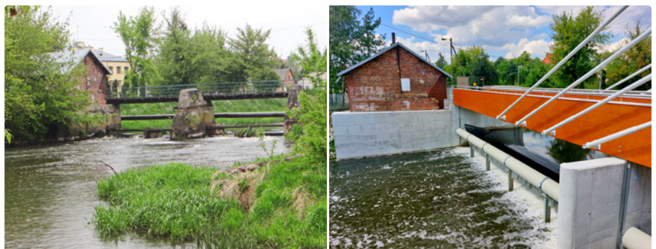
Photo 2. Weir on the Orzyc river before and after the project
