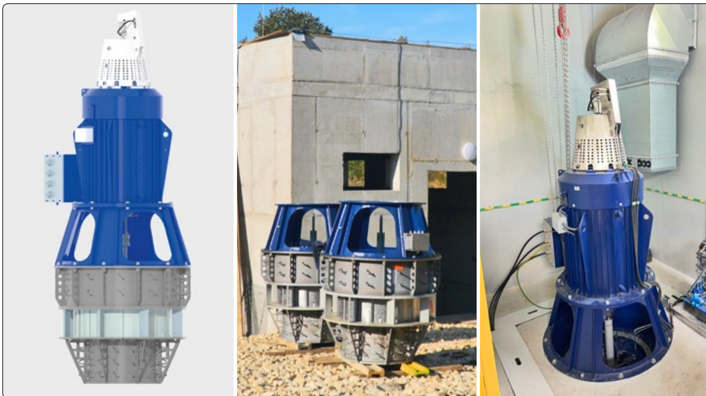
Photo 3. Kaplan turbine at different design stages, just before installation and inside the SHP building after installation
