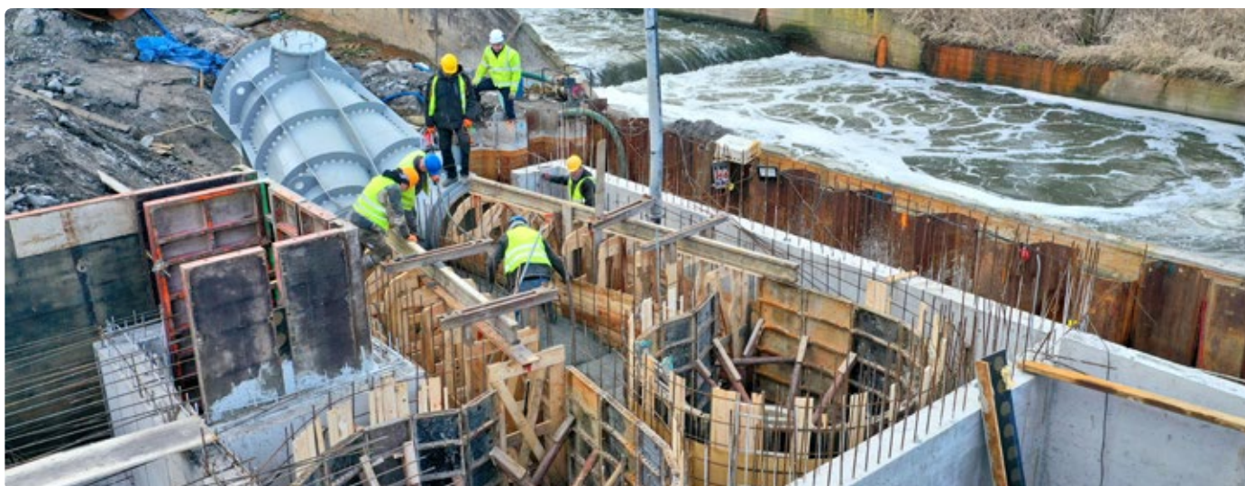
Photo 2. Preparation stage for concreting the water supply structure for the turbines
