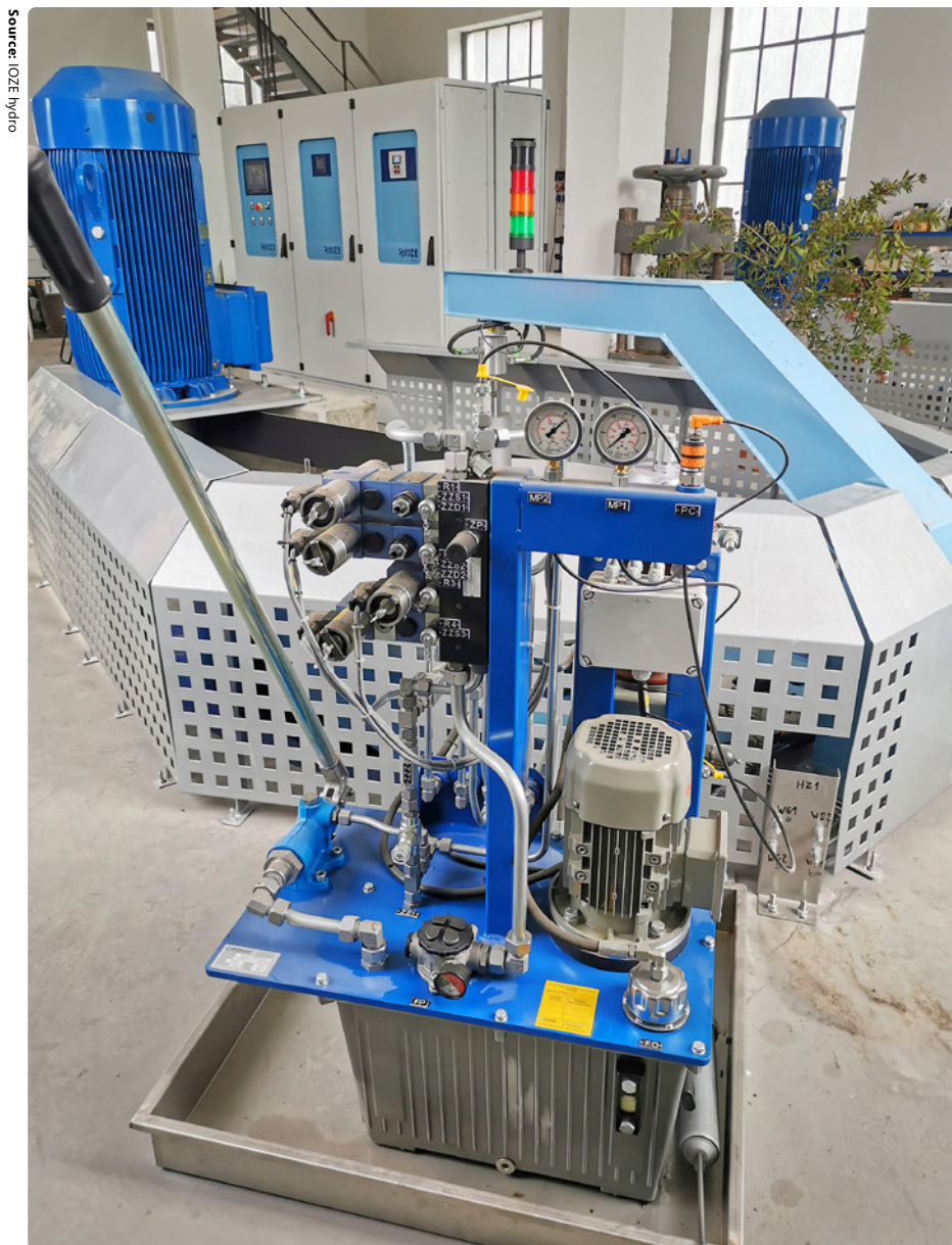
Photo 5. Interior of the machine hall after modernization
