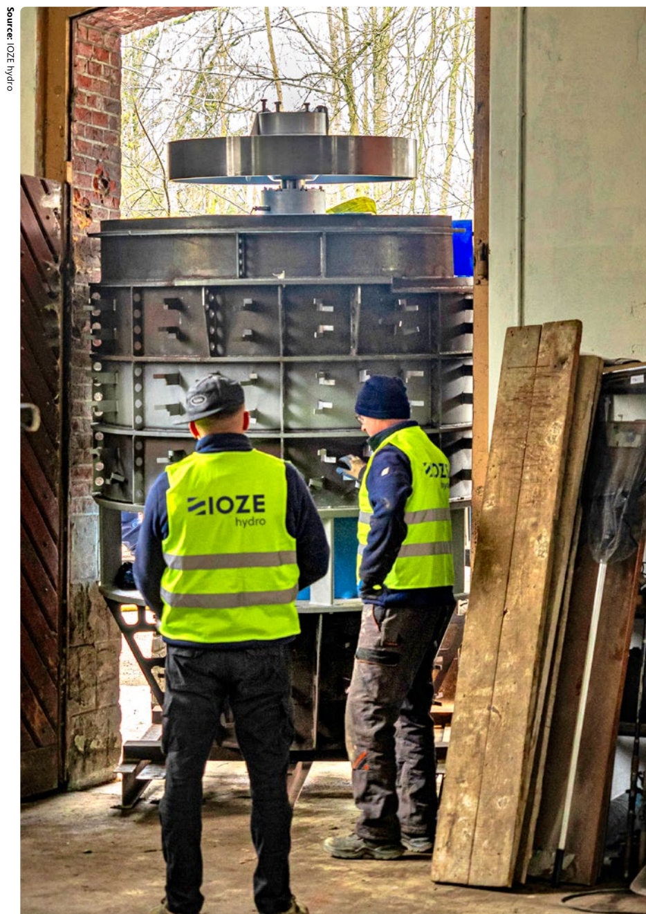
Photo: Bringing the turbines inside the watermill
