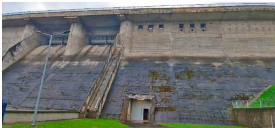
Fig. 1. A view at the Besko Dam from the tailwater's side.
